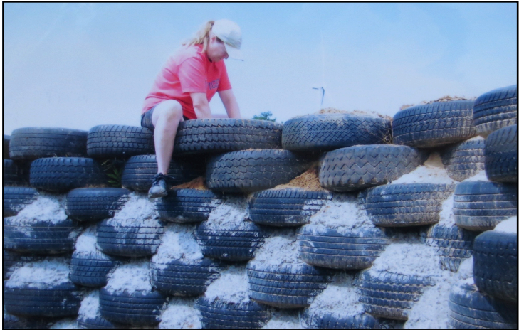
Connie works on an exterior wall made of old tires.
