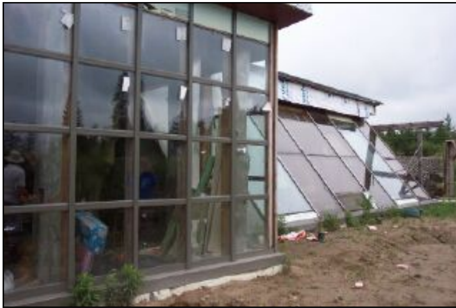
The earthship house supplies its own electricity, heat and water.
