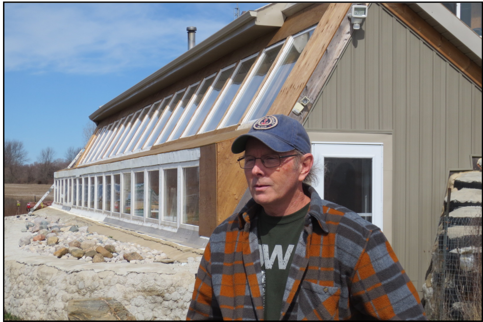
Craig Cook stands at the entrance to his earthship home near Cultus.
