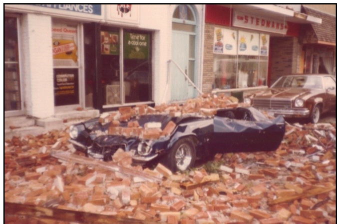
1974 Camaro was crushed by falling bricks.
